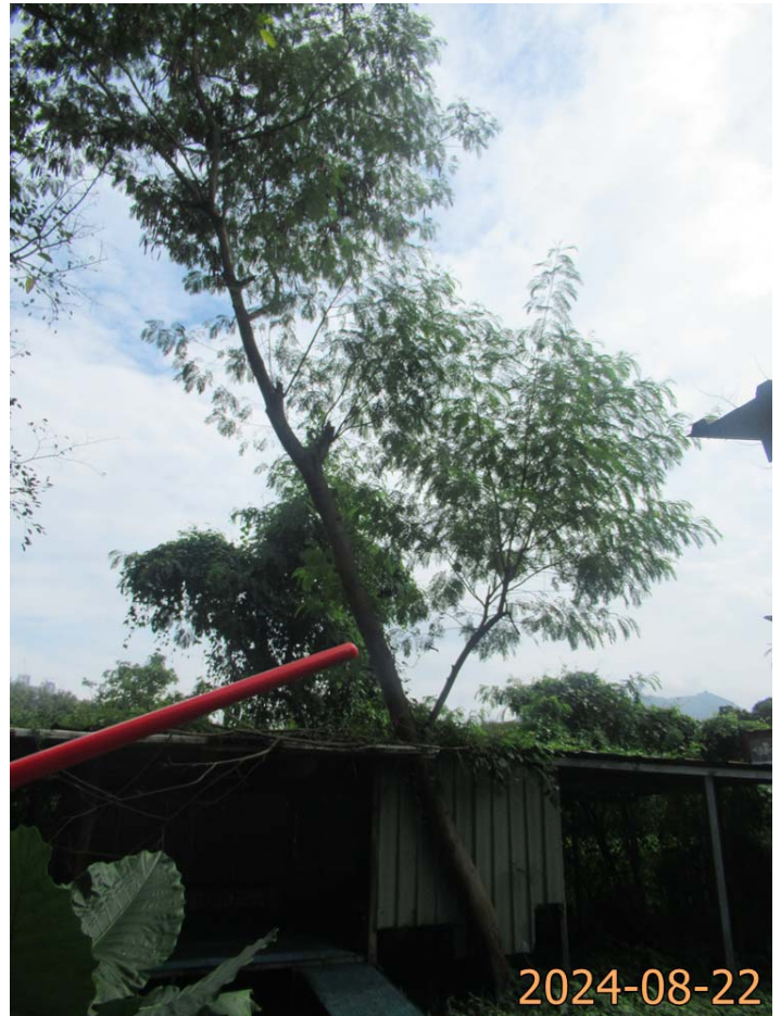
T16 (Overview) (Leaning)
